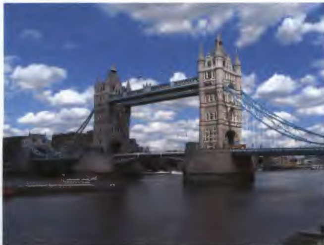
Figure 2: Tower Bridge, London. Source: Mine
