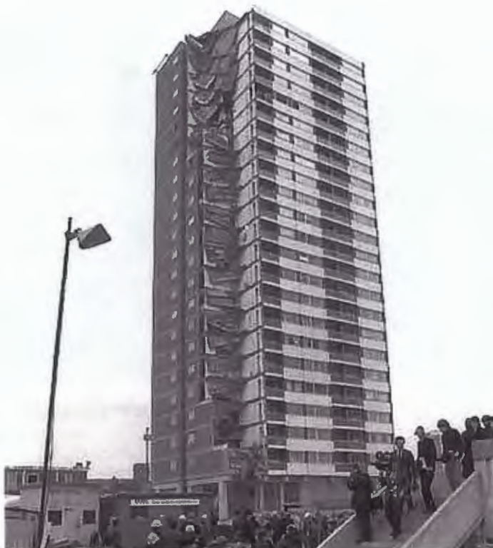
Figure 16: Ronan Point, Newham, London. Source: http://www.open2.net/modernity/3_13.htm
