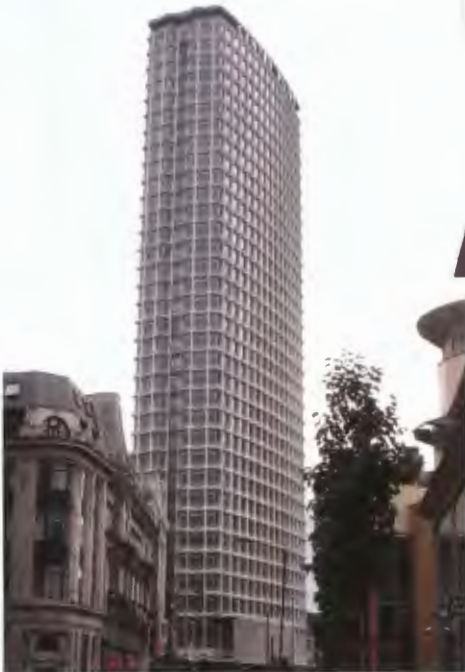
Figure 10: Centre Point, London. Source: Julia Witty
