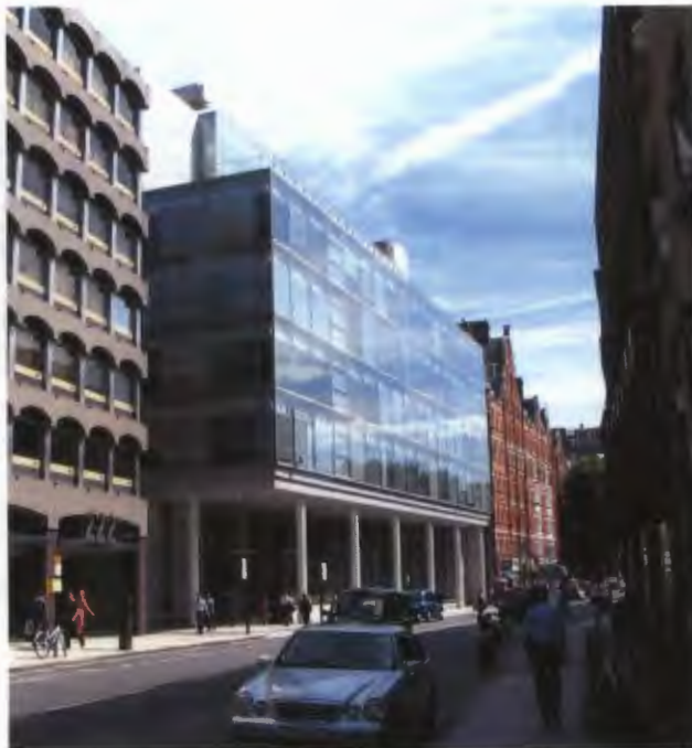
Figure 22: ITN Building, Gray's Inn Road, London. Source: Mine
