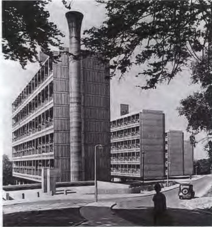
Figure 7: Alton Estate, Roehampton, Surrey. Source: http://www.open2.net/modernity/3_19.htm
