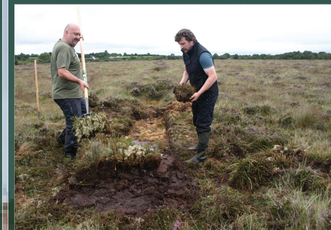
Two men construct a peat dam by hand Source: https://www.bordnamona.ie/wp-content/uploads/2021/03/WM99_RB_Restoration_Best-Practice-Guidance.pdf
