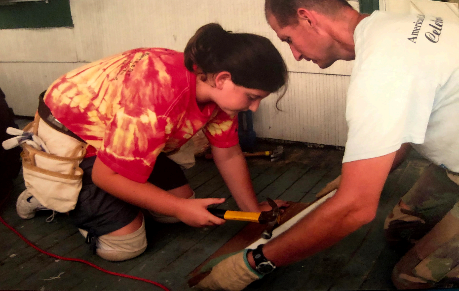
Chloe and dad doing porch repairs, 2011. Fayette County, WV.
