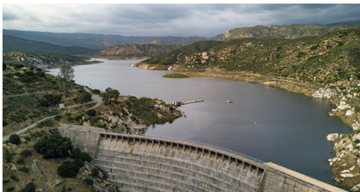
The San Vicente Dam, located 25 miles northeast of San Diego. Photo by City of San Diego.
