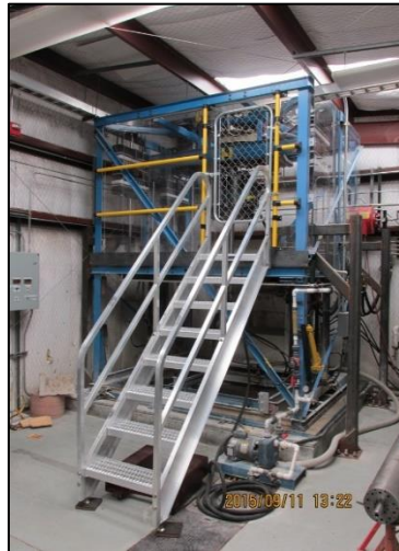
Figure 3.1. SNL Hard Rock Drilling Facility (Barnett et al., 2022)
