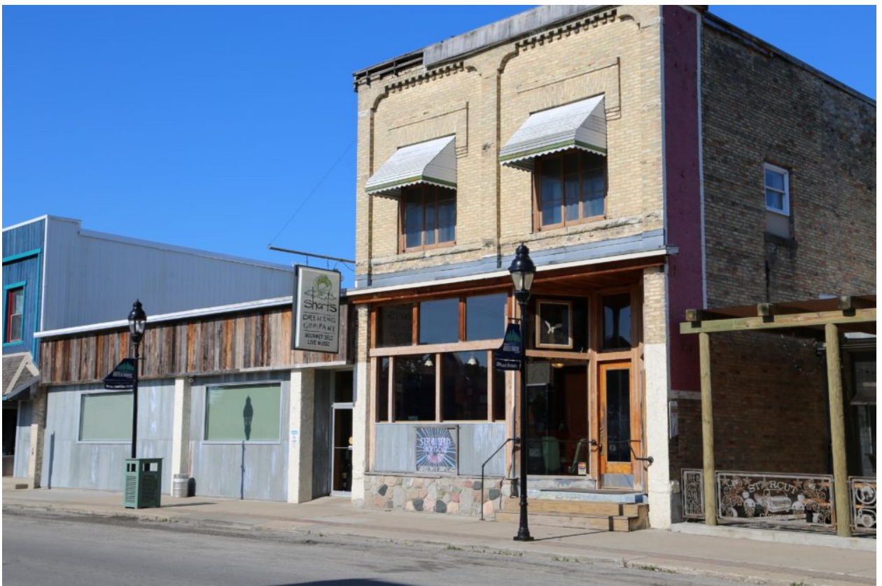
FIGURE 8: SHORT'S BREWING COMPANY'S PUB (BELLAIRE CHAMBER OF COMMERCE, N.D.)
