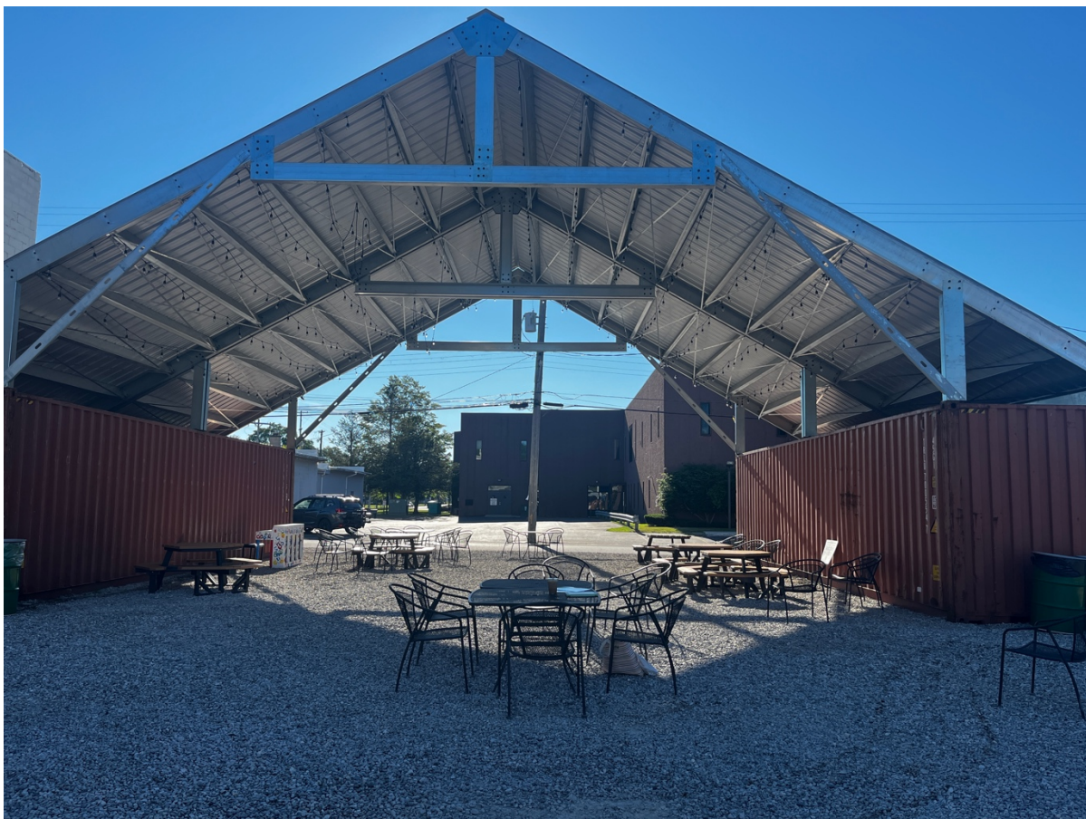
FIGURE 1: THE NEWLY INSTALLED PAVILLION OVER THE OPEN SPACE
