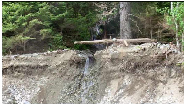
Figure 28. Photograph of FEMA DOT#18 channel from Lutak Road (June 2021).
