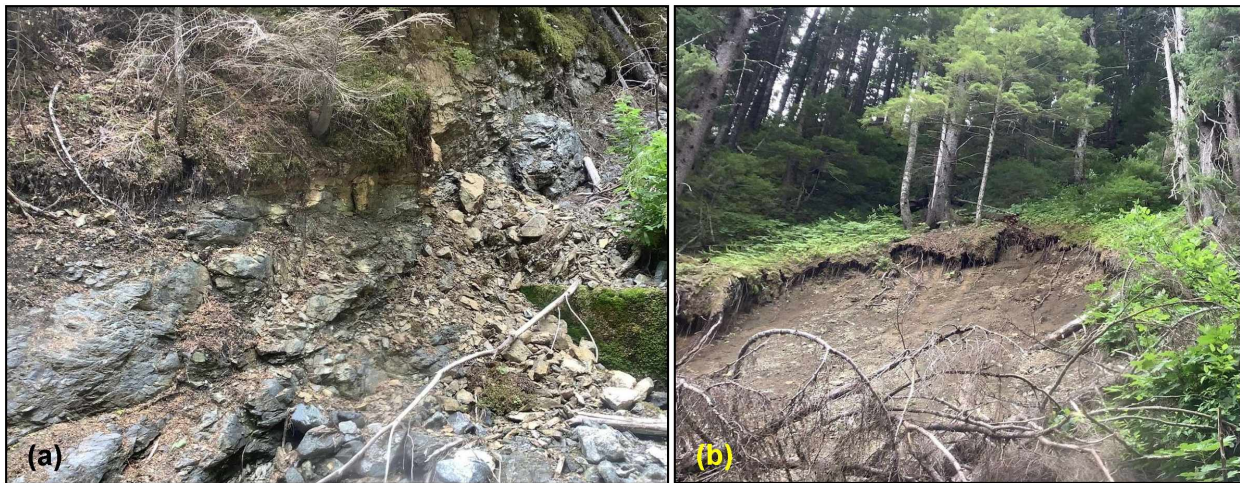
Figure 134. Photographs of upper Cunningham Creek, taken in July 2022: (a) exposed bedrock in the channel at ~126 m elev.; (b) the head scarp of one of the sources of debris for the December 2020 event (~210 m elev.).
