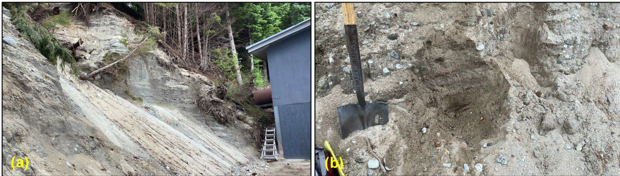
Figure 13. Photographs of the GP sand flow (June 2021 after some clearing efforts) showing: (a) alternating coarse and fine layers exposed in the left flank adjacent to the impacted corner of the house; (b) sampling location (shovel for scale).
