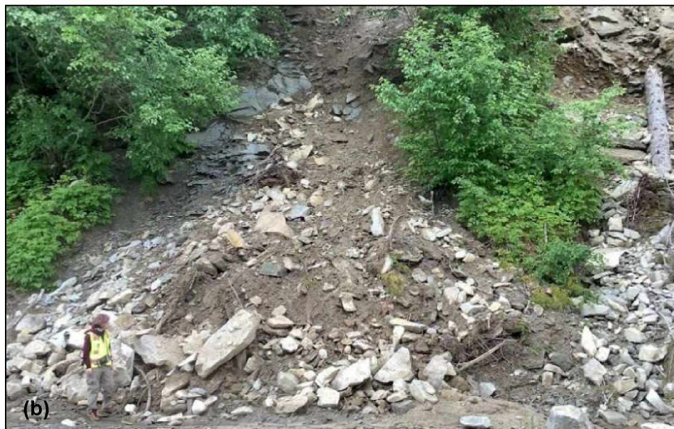
Figure 75. Views of the landslide at FEMA DOT#40 (June 2021): (a) annotated view of the left flank with exposed bedrock location; (b) right flank as visible from Lutak Road.
