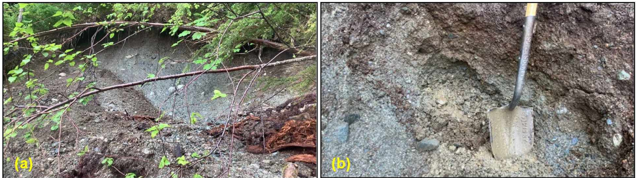
Figure 116. Photographs from the Woodshed site landslide along Lutak Road in June 2021: (a) head scarp area as seen from the property; (b) sample location, which was saturated and flowed when disturbed (shovel for scale).
