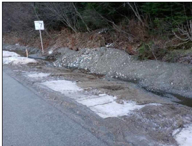
Figure 106. View of deposited material remaining in the ditch at FEMA DOT#70 after road clearing in December 2020 (photograph courtesy of ADOT&PF).
