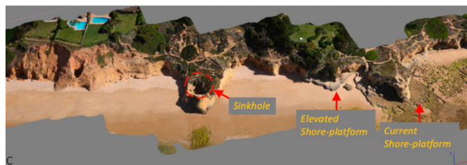
Figure 4. 3D model of the cliffs near Maria Luísa displaying sinkholes and shore platforms (STOCK 2019).
