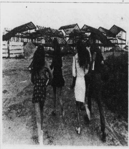
Students run to see the new Parkland building being built.
