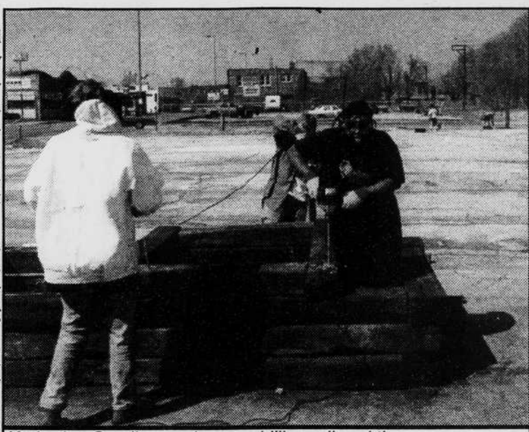
Katherine Candler, sophomore, drilling railroad ties for landscaping.
