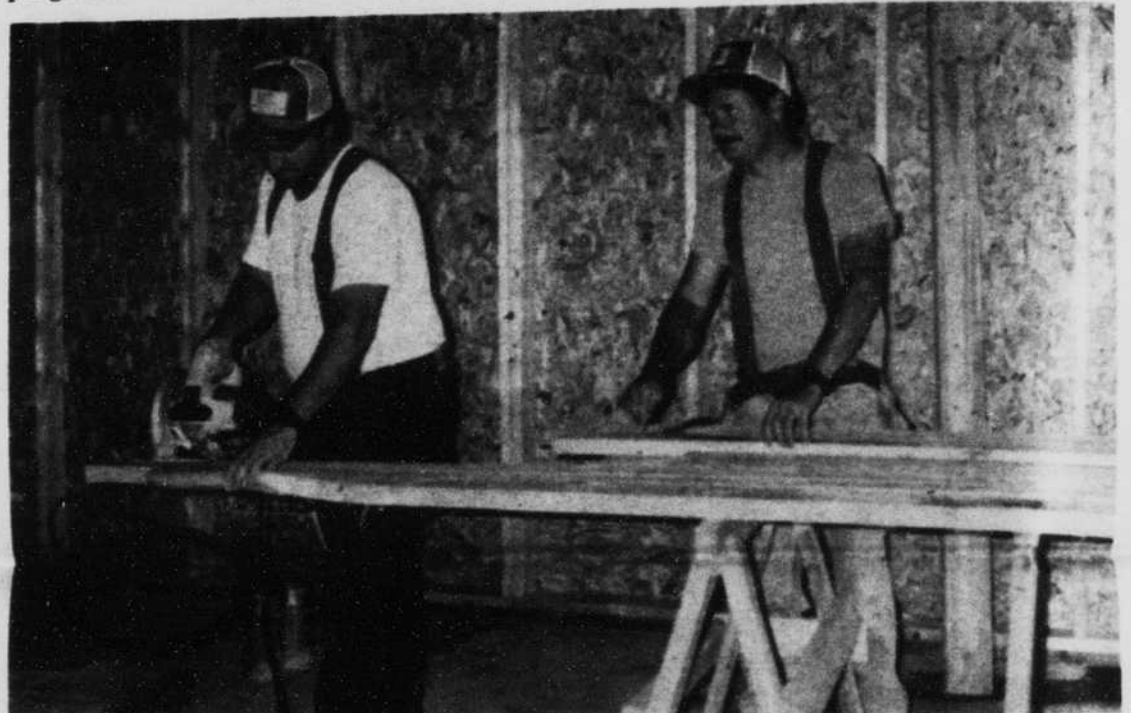
Interior work progressing
