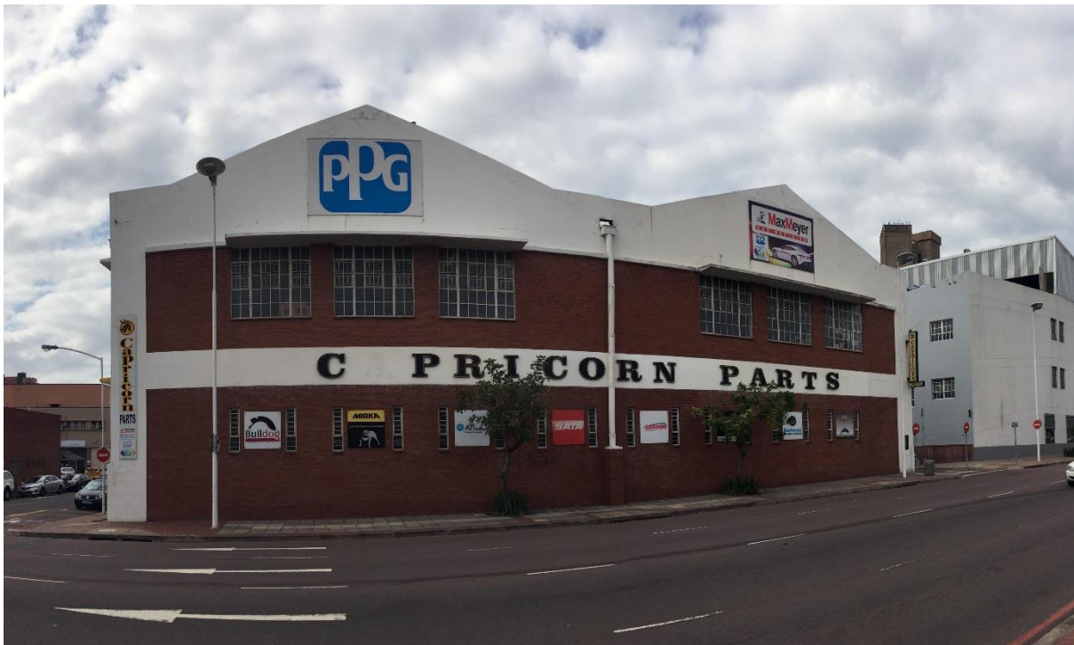
Figure 72: West elevation of the existing facebrick building on the three northern plots. (Source: Author)
