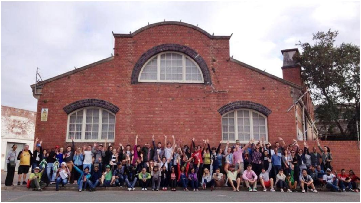
Figure 49: Florence Nzama Street elevation. (Source: BESETDurban)
