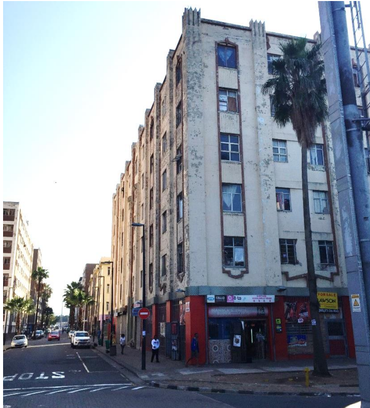
Figure 62: An example of the condition of many of the buildings in the Durban inner city, this one near Albert Park. (Source: Author).
