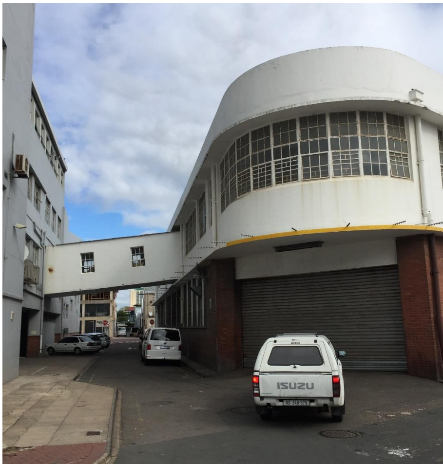
Figure 74: The existing sky bridge that links the two existing buildings. (Source: Author)
