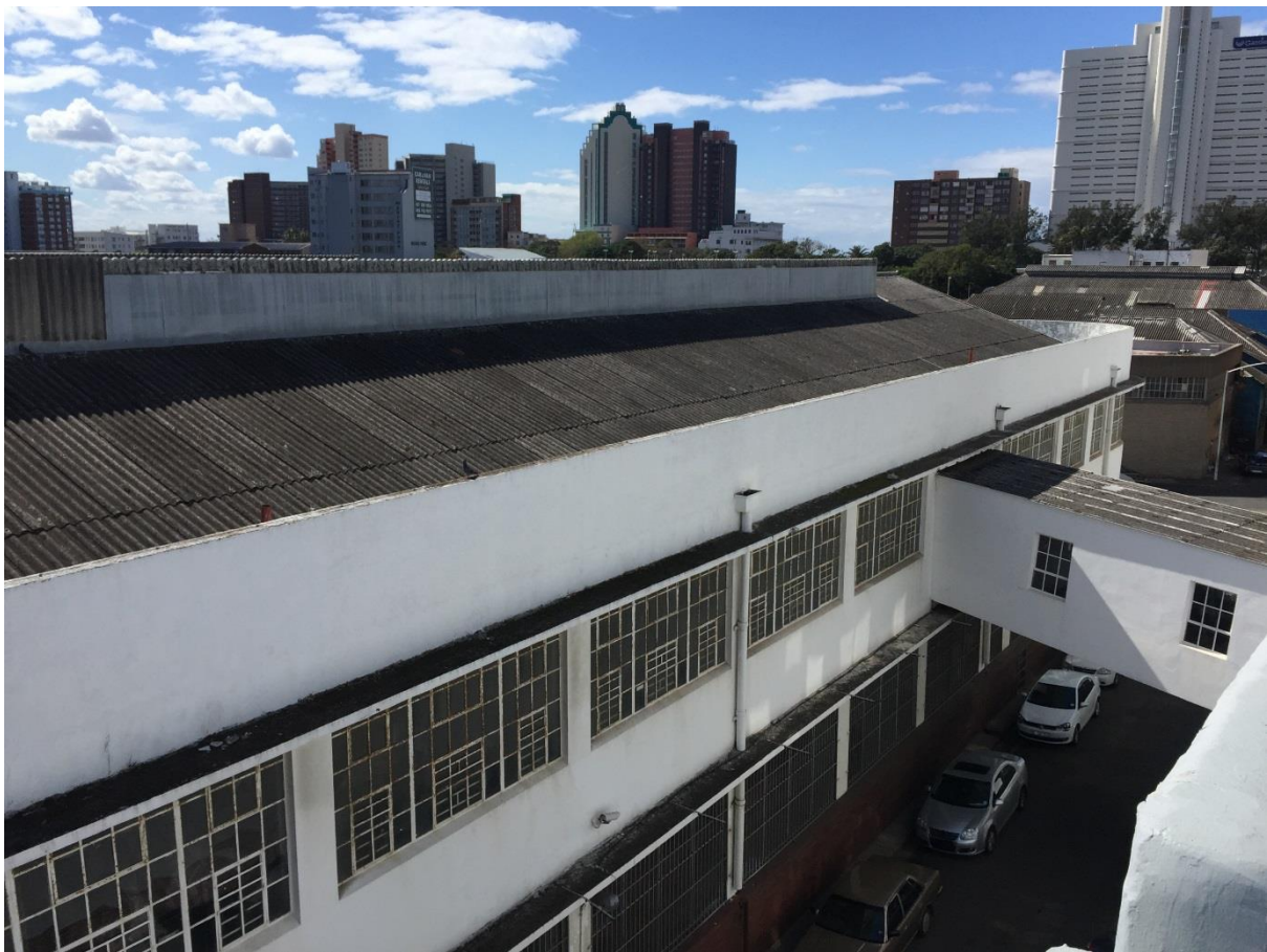
Figure 79: Existing fibre cement roof of Capricorn Parts. (Source: Author)
