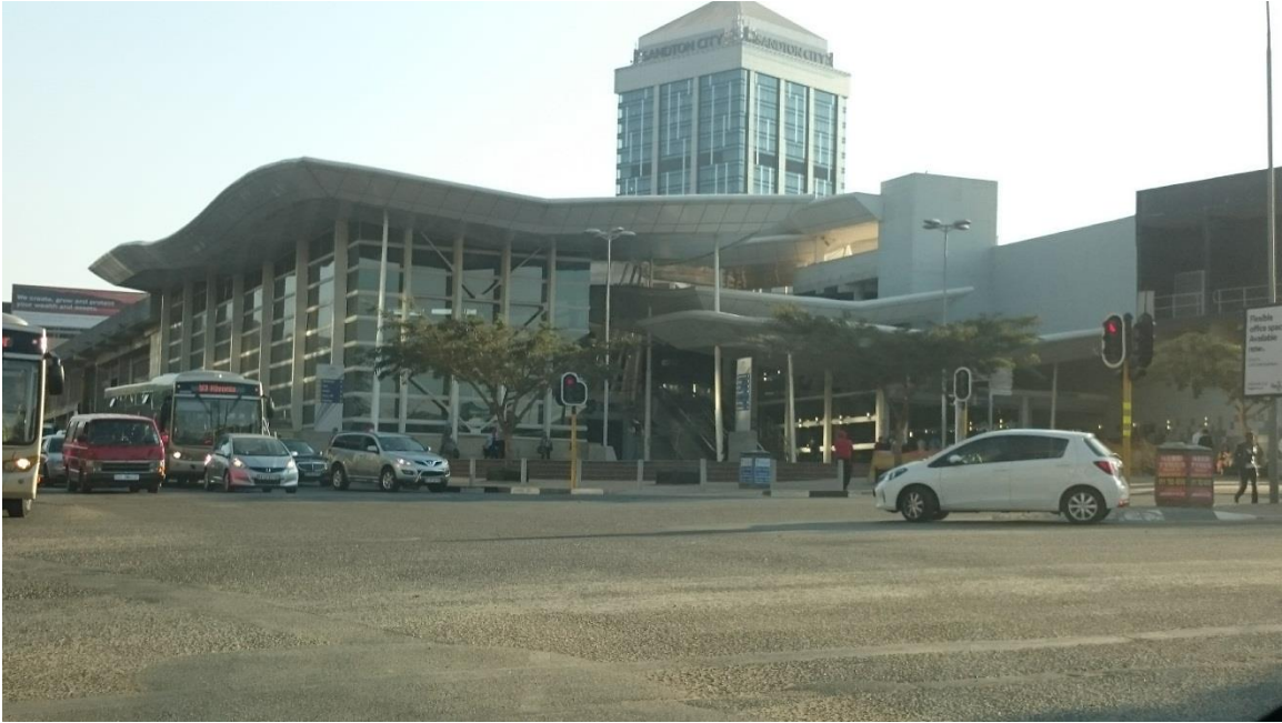
Plate 6-16. Wavy roof celebrates entrance as at the Sandton Station. Source: Author
