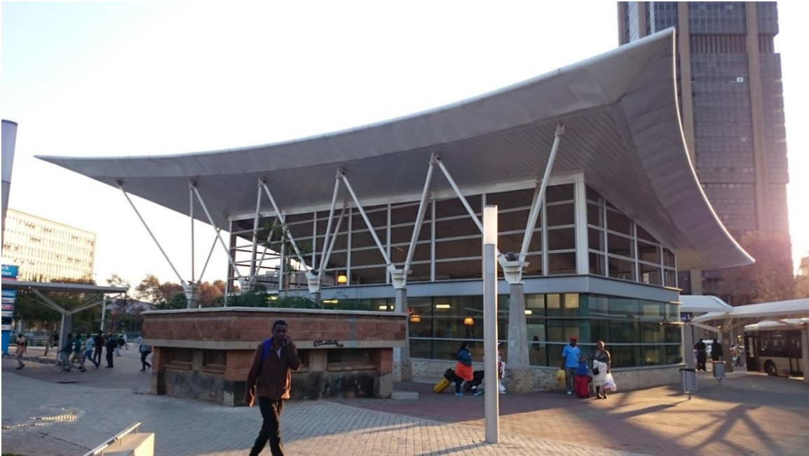
Plate 6-21. Station entrance at Park station in central Johannesburg. Source: Author
