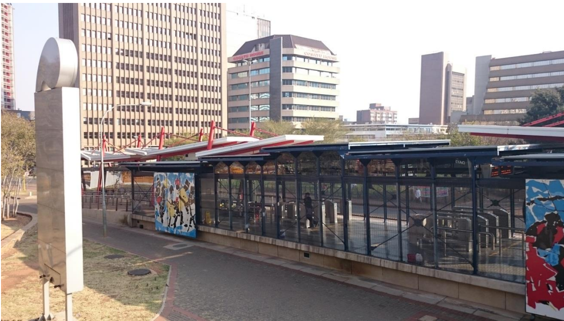
Plate 6-12, 6-13, 6-14. The use of art and sculpture to enhance architectural aesthetics. Building structure houses advanced ticket collection systems. Source: Author
