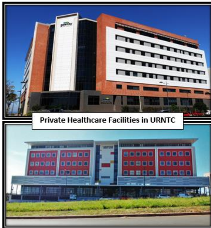
Photo 12: Gateway Private Hospital & Medstone Medical Centre
