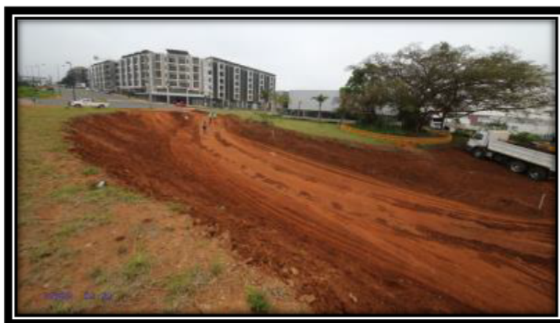
Photo 16: N2 & Cornubia link, URNTC - Earthworks
