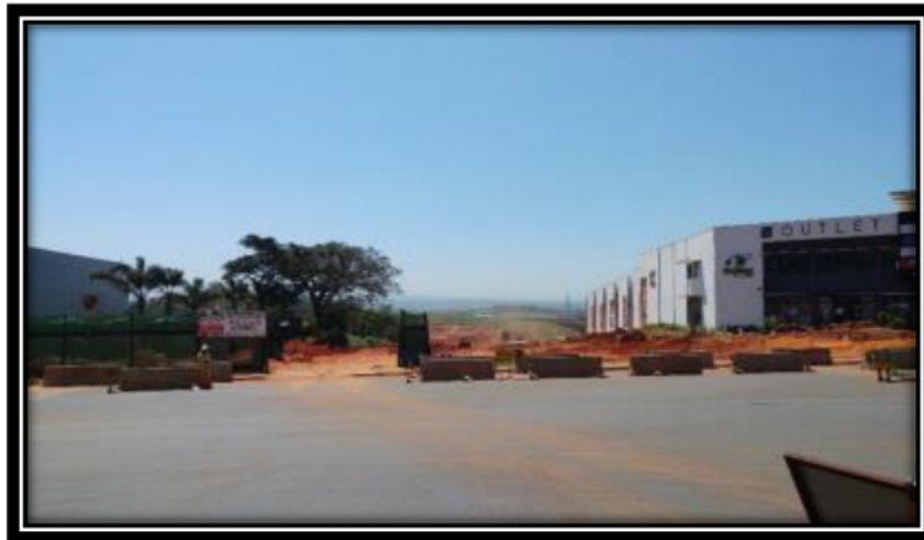
Photo 17: IRPTN C9 route construction site within URNTC
