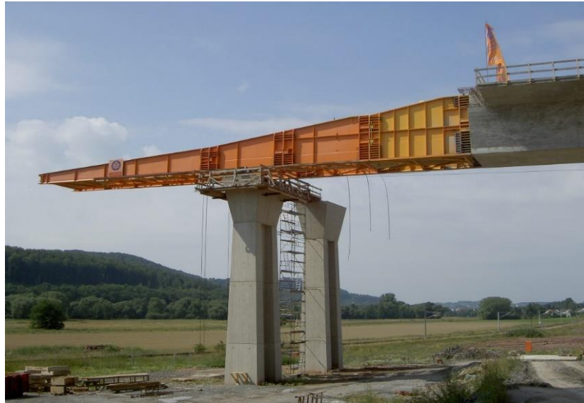
Figure 1.5. Incrementally-launched bridge construction (Valley Bridge Coburg)
