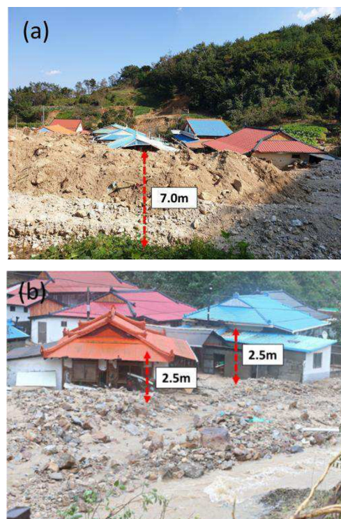
Fig. 5. The situation at the time of the damaged and height of inundation trace. (a) : Site A, (b) : Site B.
