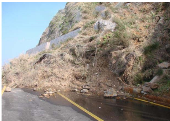
Fig. 1. Debris flow in SS 113 km 84+800 in the municipality of Gioiosa Marea (ME) in December 2011.
