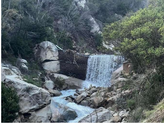
Fig.5. Filled SVX barrier after debris flow event (Photo: Pat McElroy).
