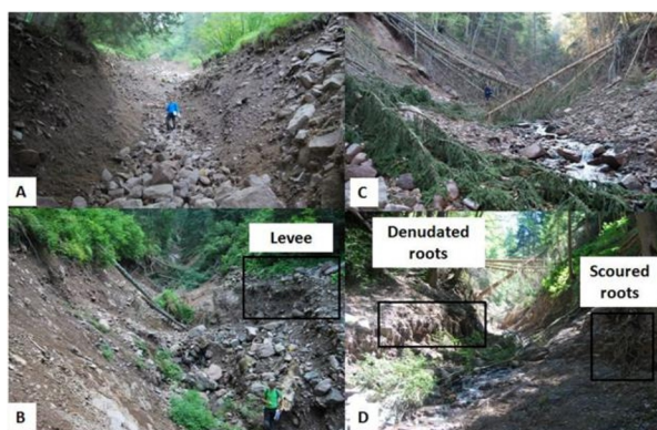
Fig. 2. Photos of the debris-flow torrents in the upper reaches (A), middle reaches (B), and lower reaches (C and D); field traces are highlighted in B and D.
