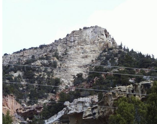
Fig. 4. Study area 3, subsidence contours, cell locations and escarpment failure zones shown in red (top), observed failure pattern (bottom).
