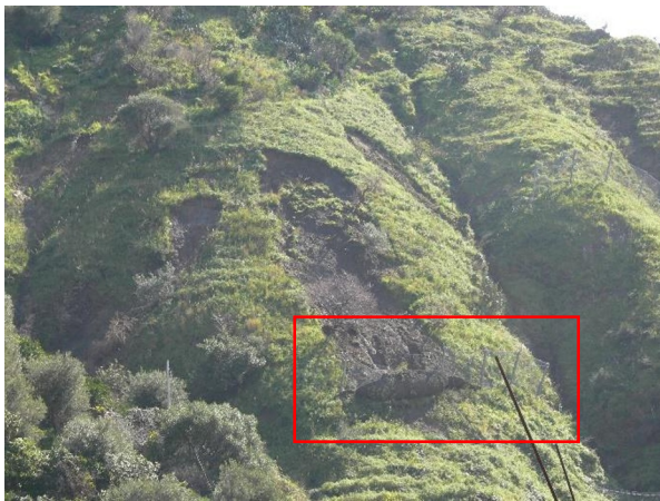
Fig. 3. Partially filled shallow landslide / hillslope debris flow barrier SL-150 (red rectangle) with the starting zone above the structure.
