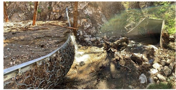
Fig. 2. Filled debris flow barrier with inlet downstream.
