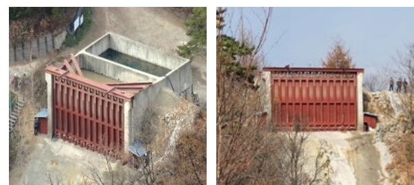
Fig. 4. Debris flow initiation facility at top view (left) and front view (right).
