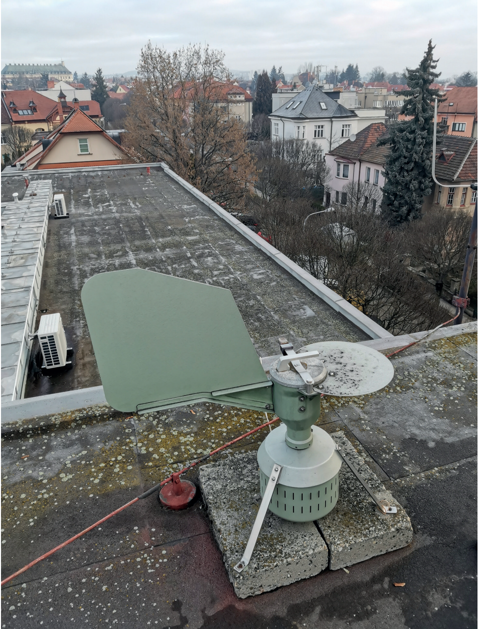
Figure 1. 7-day volumetric air sampler (Burkard Manufacturing Co Ltd, Hertfordshire, UK) in Brno (Czechia) installed on the roof of the University hospital, 15 m above ground to ensure landscape-scale monitoring. Photo credit for Aneta Lukačevićová.
