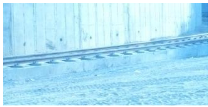
Direct fixation slab track
