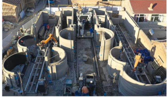
FARMHOUSE - TSINGHUA UNIVERSITY 3D concrete printing construction with 62,4% reduction in human resources. Xu et. al, 2022
