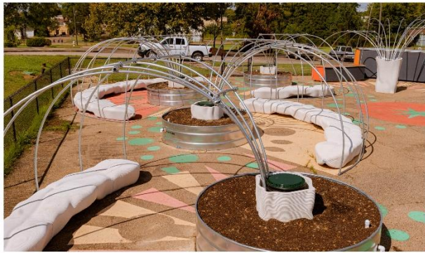
LEARNING GARDEN - MISSISSIPPI STATE UNIV. 3D printed benches and pipe "stems" for Galloway Elementary in Jackson, MS.
