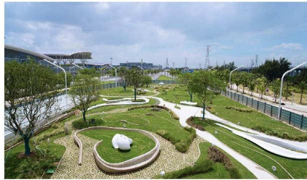
PARK - TSINGHUA UNIVERSITY 3D printed park in Shenzhen, China with benches, sculptures, paving and retaining walls.
