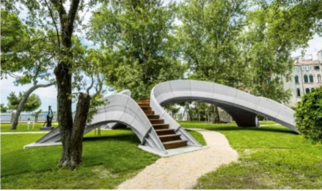
STRIATUS BRIDGE - ETH ZURICH Footbridge designed as compression-only structure without reinforcement. Bhooshan et. al, 2022
