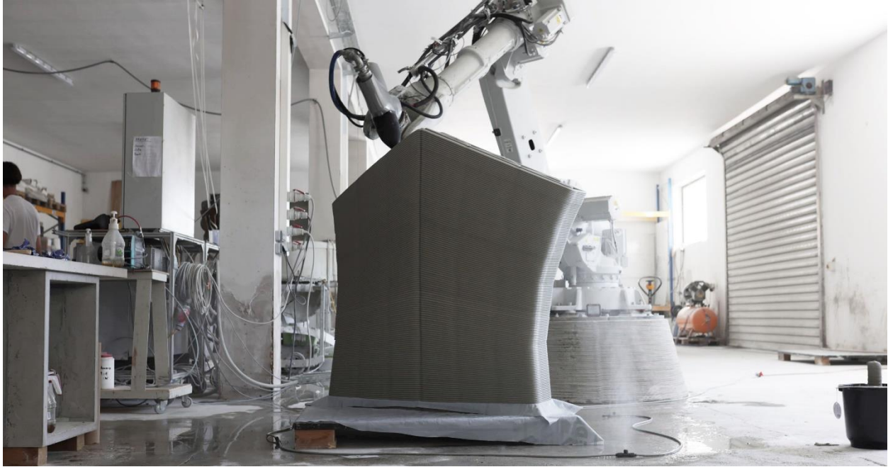
Figure 2.24 A typical robotic arm set up with incremental3D, printing modules for the Striatu bridge
