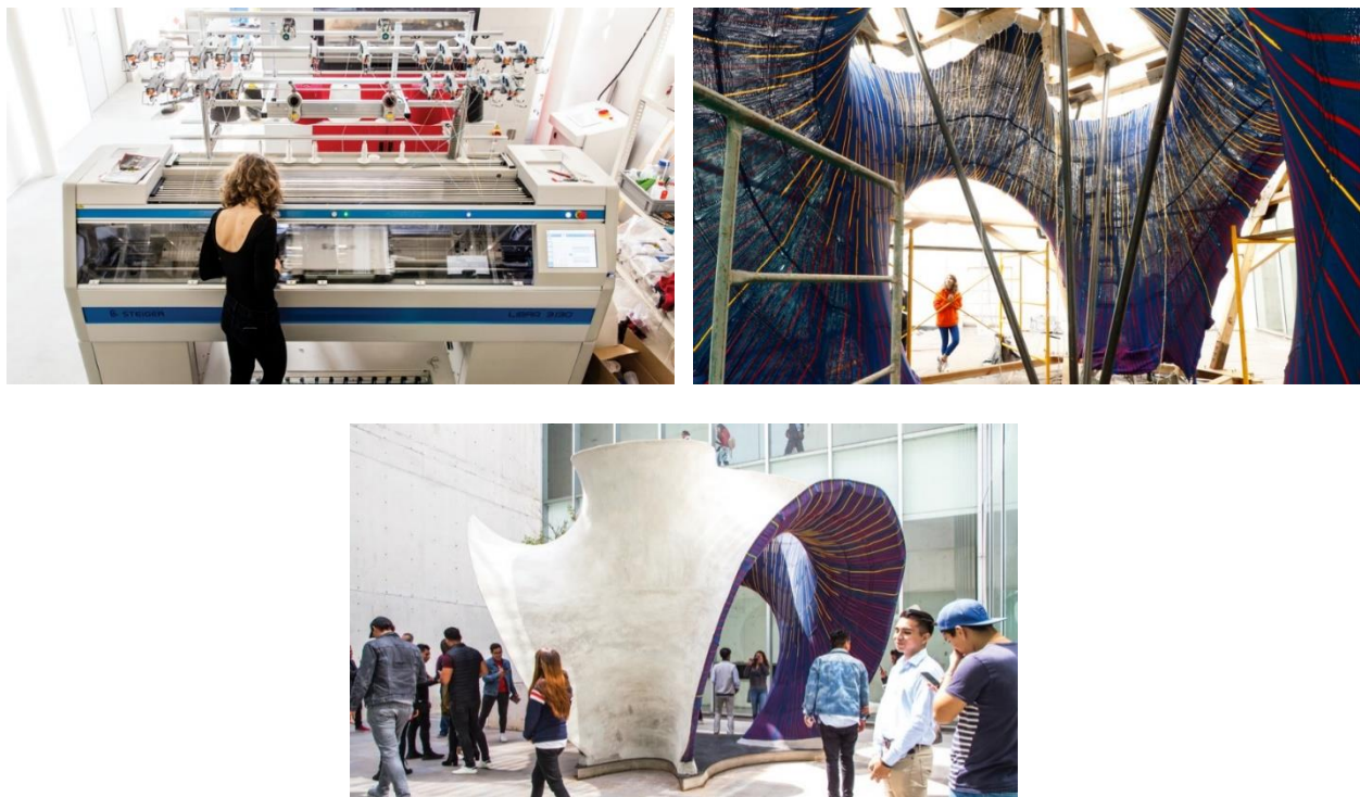
Figure 2.10 KnitCandela, Mexico City, 2018, Product of KnitCrete flexible knitted textile formwork
