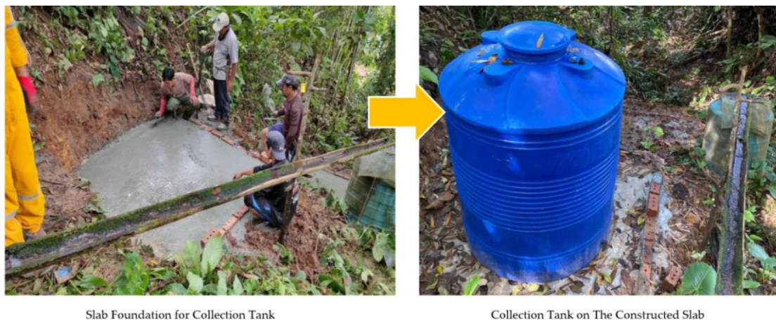
Fig. 6 - Construction of collection/ header tank station at water intake station
