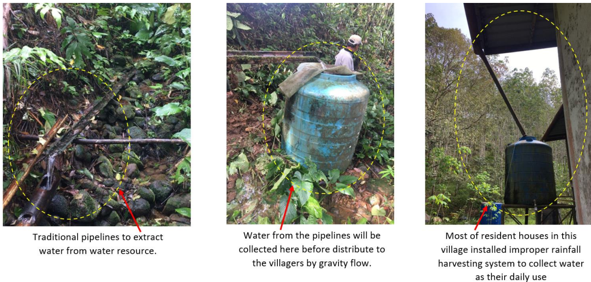
Fig. 1 - The existing water collection system in Kampung Bongol, Sabah
