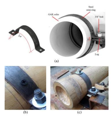
Fig. 6 - Steel clamping configurations for bamboo culm truss connections [26]
