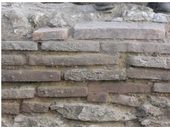
Fig. 17 Opus testaceum of Viminacium thermae wall. Photo by the author.
