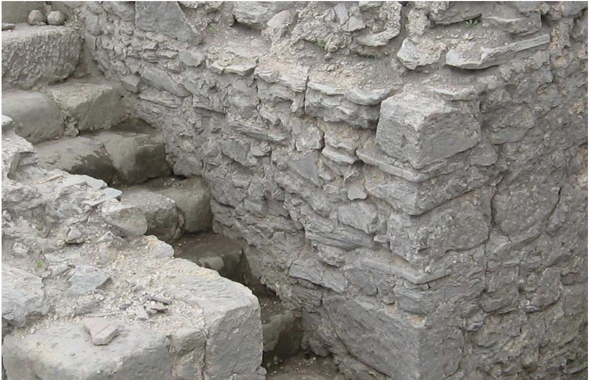
Fig. 25 Opus incertum in the rooms outside the arena of the amphitheatre with visible blocks of limestone on the wall corners. Photo by the author.
