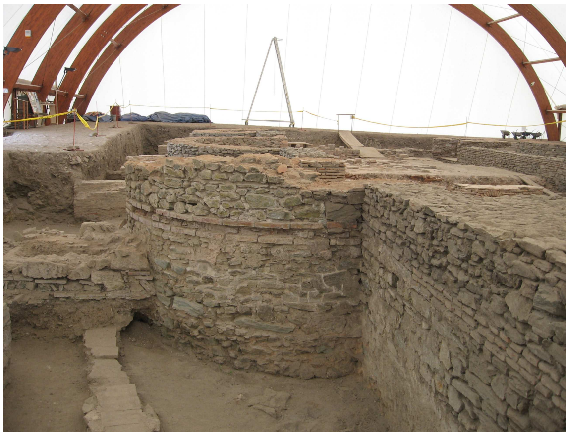
Fig. 32 Opus incertum mixtum in the walls of Viminacium thermae. Photo documentation of the Project Viminacium, Archaeological Institute Belgrade.
