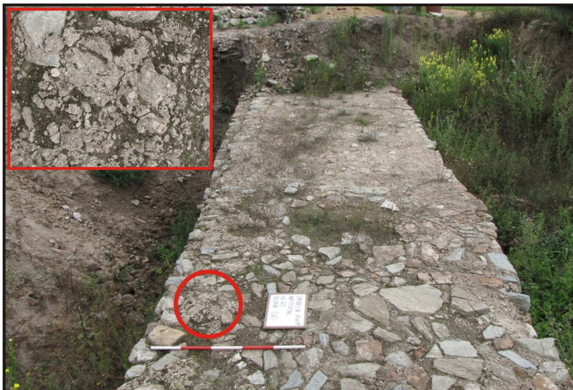
Fig. 23 Wall of the city rampart with the picture of the hard lime mortar without addition of brick. Photo documentation of the Project Viminacium, Archaeological Institute Belgrade.
