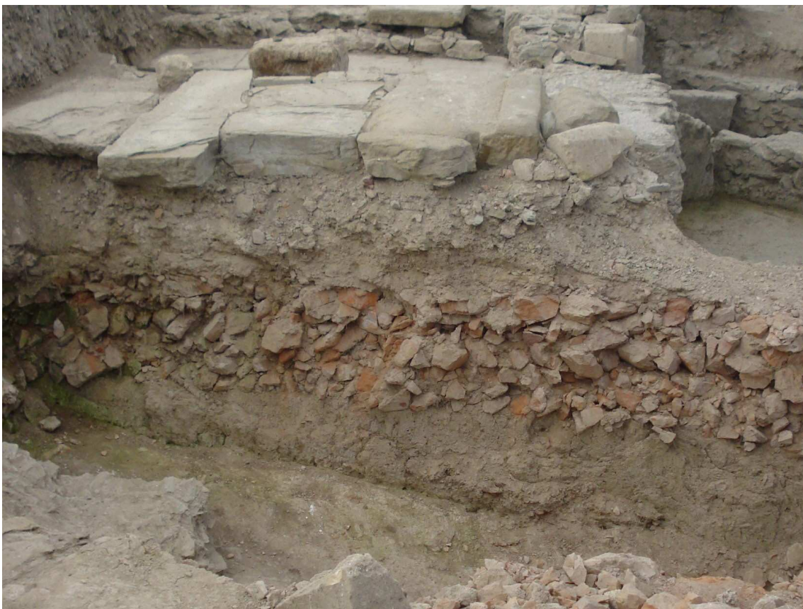
Fig. 16 Substructure of the road entering the northern gate of the legionary fortress. Photo by the author
