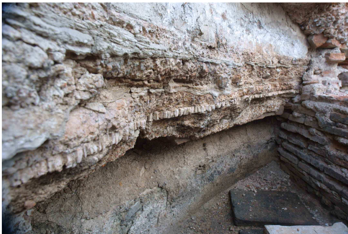
Fig. 22 Lime mortar for floor layers of the thermae with the addition of brick. Photo documentation of the Project Viminacium, Archaeological Institute Belgrade.
