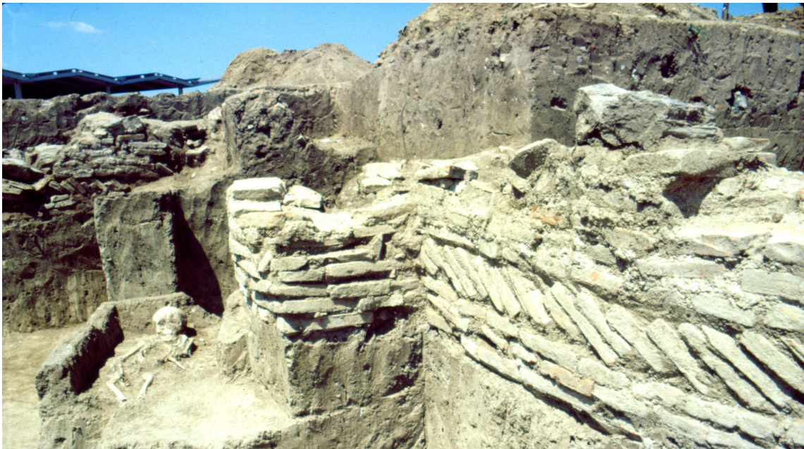
Fig. 36 Opus spicatum in the wall of the tomb. Photo-documentation of the Republic Institute for the Protection of Monuments.
