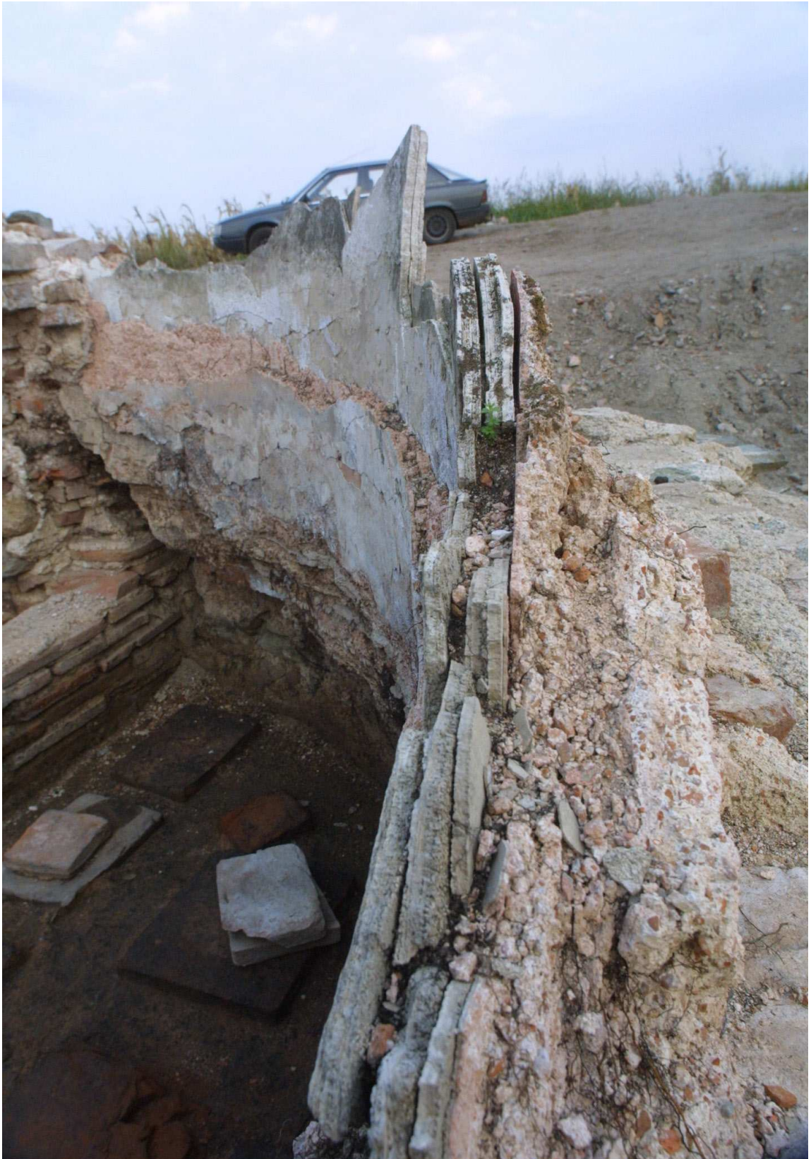
Fig. 21 Lime mortar for plastering of the thermae walls with the addition of brick. Photo documentation of the Project Viminacium, Archaeological Institute Belgrade.
