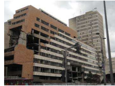
Figure 3 - Building B, corner of Nemanjina St. and Kneza Miloša St.
