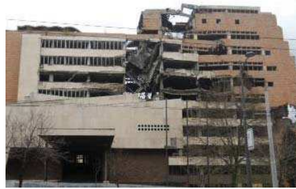
Figure 2 - Building A, facade to Kneza Miloša St.
