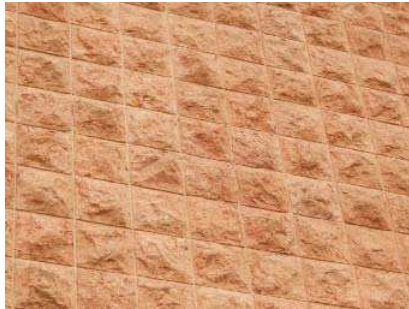
Figure 11 - Preserved wall surface of "Koral" on building B
