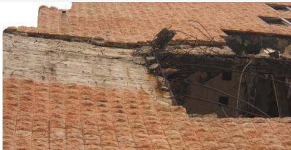
Figure 4 – Big wall surfaces of red stone built simultaneously with casting of concrete
