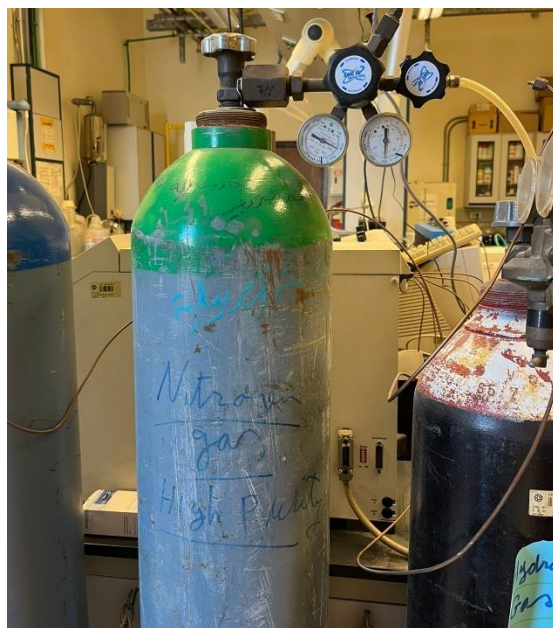
Figure 3-12: Nitrogen Gas Cylinder
