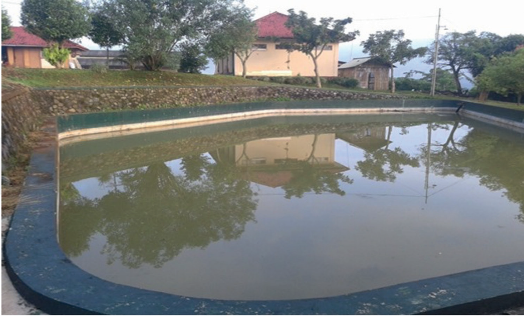
Figure 6. Micro and semipermanent rainwater harvesting ponds at Pakuwon Agrosience Park, in Sukabumi, West Java.
