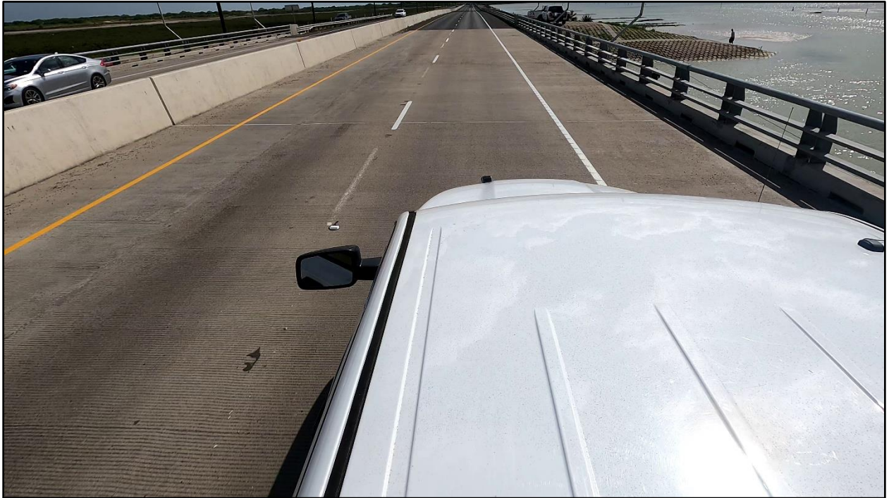
Figure 5. Example section of concrete traffic barrier (median barrier pictured) and T2P railing (side barriers pictured) with metal poles extensions (which were kept through the transition from concrete to T2P). The road pictured is Texas State Highway 48 in Cameron County, Texas, USA.
