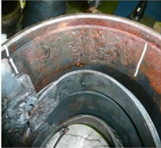
Figure 7: L-4 spalled inboard cup believed to be responsible for derailment [10]
