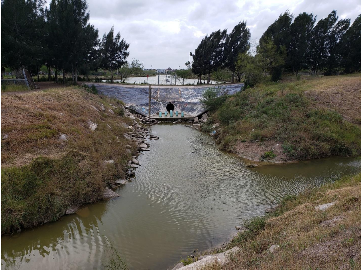
Figure 21: Drainage structure at a Resaca in Brownsville, TX
