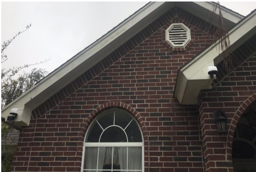
Figure 4.2: Installation photo of the pre-study sample in site W1.
