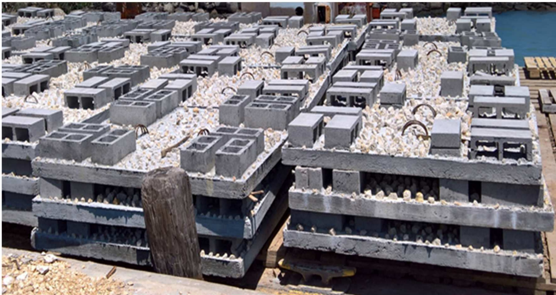
Figure 4: Concrete low-profile modules used in the experimental reef area in the Rio Grande Valley artificial reef. ~0.5 m of vertical relief
