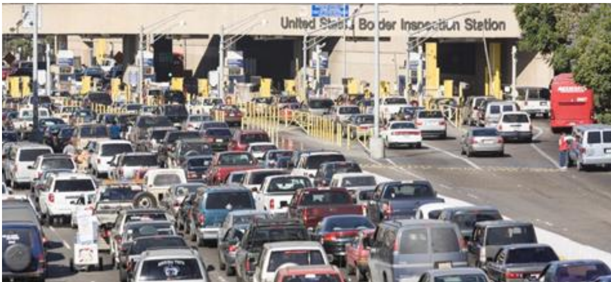
Figure 2: Aerial photography of a POE station between the U.S. and Mexico (by Arthur Greenberg/ Shutterstock)
