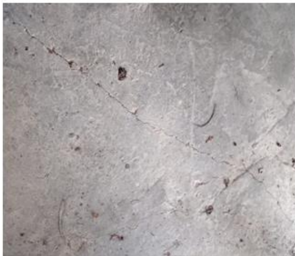
Fig.2: Plastic Shrinkage (Ghourchian et al., 2017)
