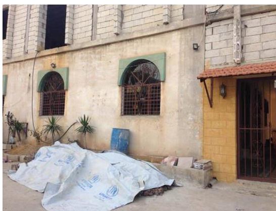
UNHCR tarp covering construction material in front of al-Bahsa new mosque in Akkar, North Lebanon. March 2018.
