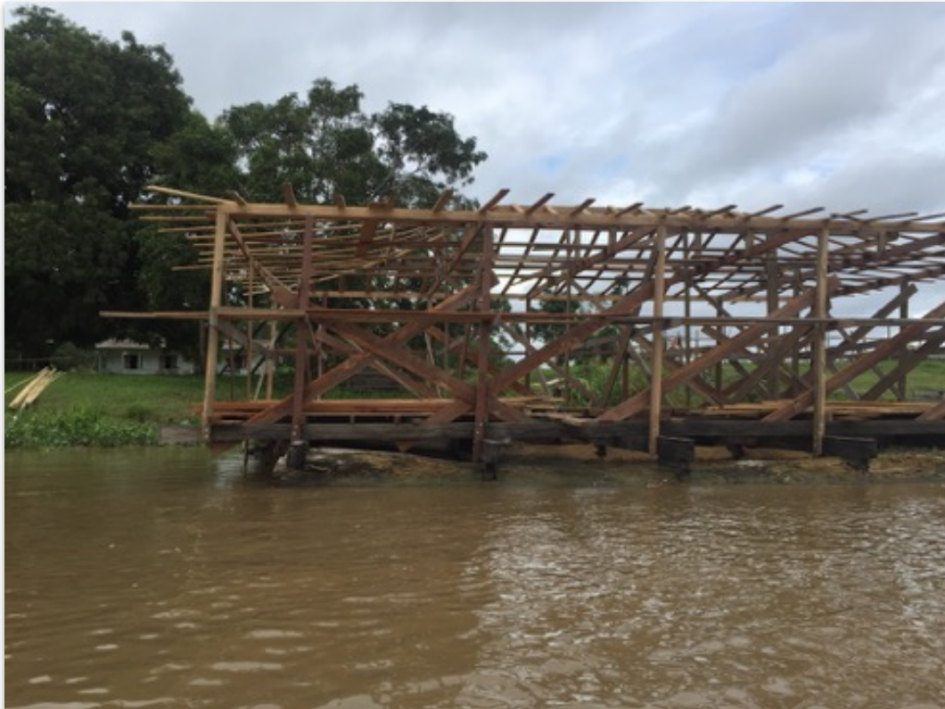
Figure 62. Unfinished floating house in Careiro da Várzea, Amazonas. Source: Personal Collection (2018).
