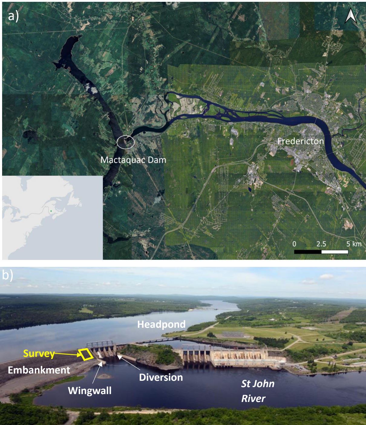
Figure 4.1: Mactaquac Dam. a) The location of Mactaquac Dam within Canada and its more localised location in New Brunswick, Canada (45.95°N, 66.87°W) (Google Earth, 2023). b) An annotated photograph captured of Mactaquac Dam, showing the features of the dam and the area where the ERT survey is located (modified from Butler & Boulay, 2020).
