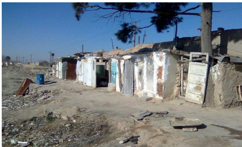
Figure 6. Illegal housing at Farahzad in the north of the Tehran municipality (Photo: Zahra Hosseini).
