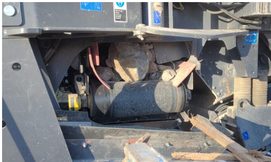
Figure 30. Relatively large natural stone jammed between the oversize conveyor and plant frame, preventing conveyor operation.
