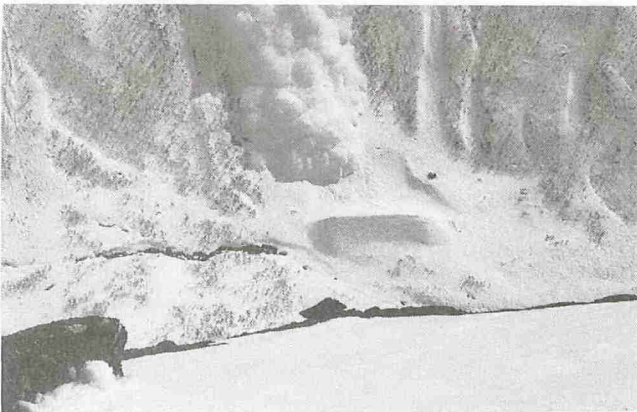
Fig. 5 The Ryggfonn avalanche as it passes over the retaining dam
