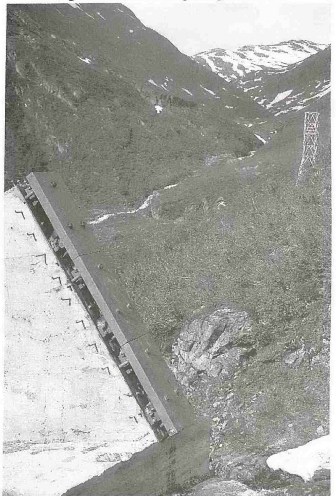
Fig. 4 Concrete tower with pressure transducers in Ryggfonn
