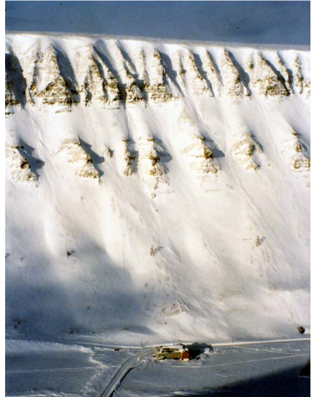
Fig. 5 The community centre and restaurant Huset is exposed to avalanches and rockfall. Cornices are built along the rim. Rockslides might be a future problem. Photo E. Hestnes.
