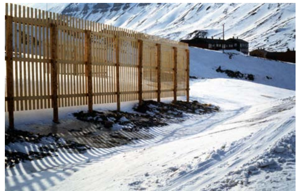
Fig.11 Snow fence before strengthening the construction and adjusting the ground clearance. Photo E. Hestnes
