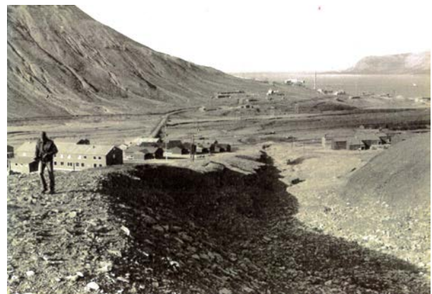
Fig. 9a The small slushflow 14 June 1989 climbed the old guiding dam and damaged a private home. It went on to the floodplain breaking the water and heating pipes and closing three roads. Photo K. Anthonsen
