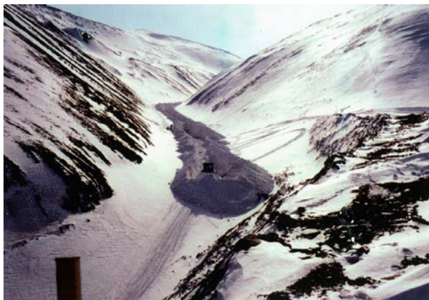
Fig. 6 Opening of the drainage channel in Vannledningsdalen by bulldozer before periods of runoff. Photo E. Hestnes
