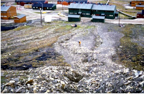
Fig.4 Houses in road 226 are built on old debris and debris deposited in 1972, and hit by a debris flow in 1981. Photo E. Hestnes.
