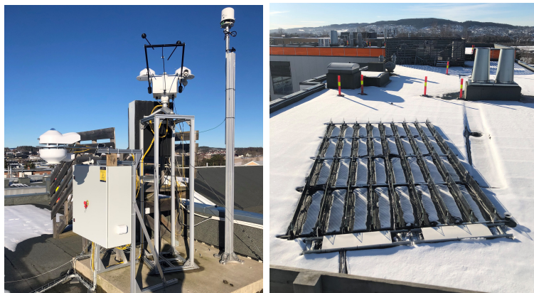
Figure 28: Objects north (left) and south (right) of the PV system.
