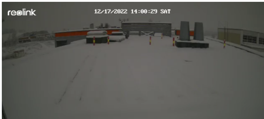
Figure 38: A picture of the test site taken by a webcam from the north the 17 th of December 2022 at 2:00 PM.
