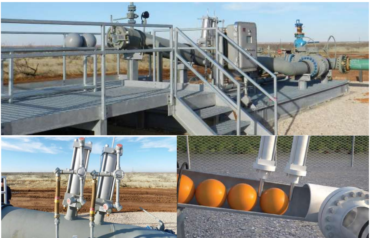
Figure 11. Spherical pigs and their launching unit on one of Tulsa’s fields Source: “The re-emergence of spherical pigs” by Larry Payne [11].
