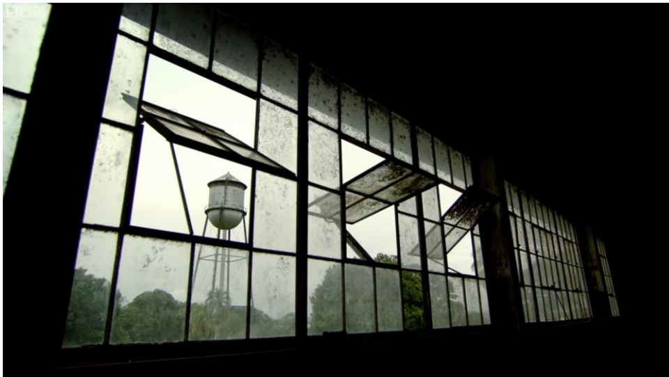
The water tower seen from inside the sawmill (Palin, 2014).
