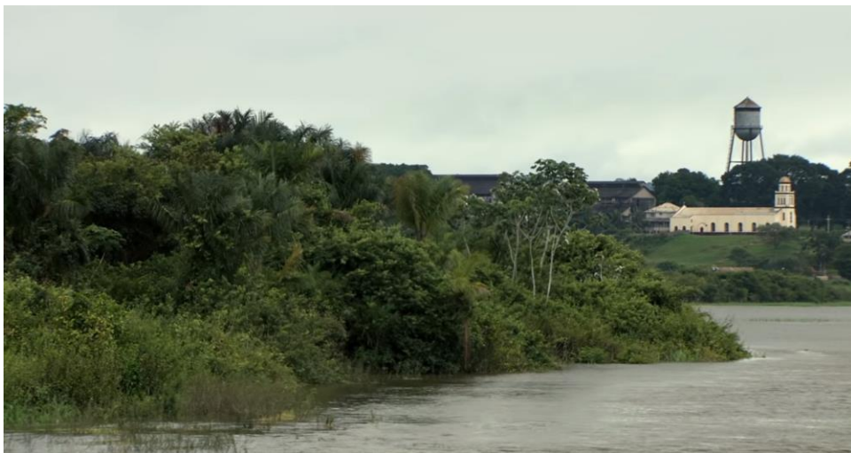
The water tower peaking up behind the church and some houses near the riverbank (Palin, 2014)
