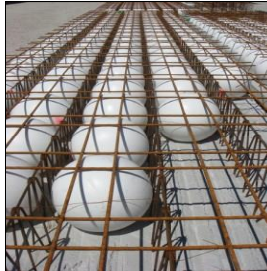
Figure 25: Bubble Deck (Constructor, 2023)
