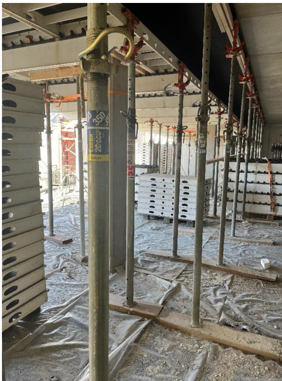
Figure 27: Temporary struts
