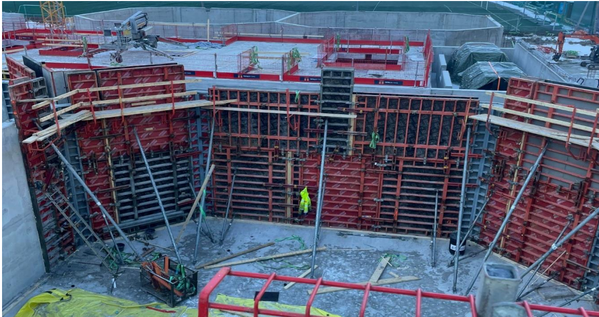
Figure 5: System formwork used by Total Betong AS
