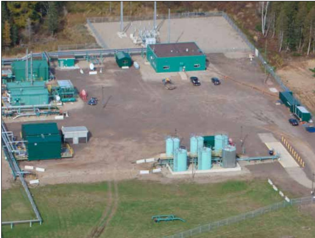
Figure 3.3 Corridor Resources Drill Site near Sussex New Brunswick
